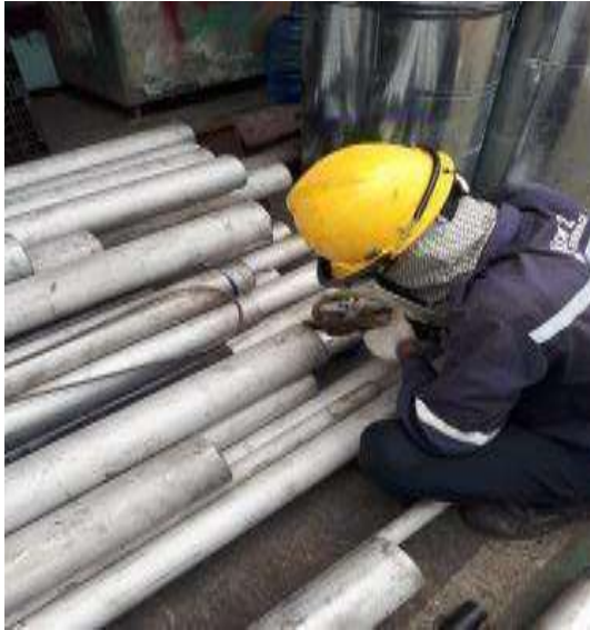
Pipe beveling and spool pipe fabrication at Gajah Tunggal project
