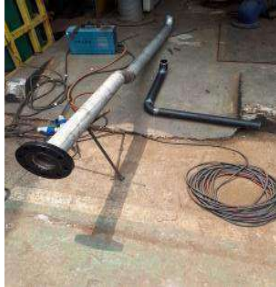
Pipe beveling and spool pipe fabrication at Gajah Tunggal project
