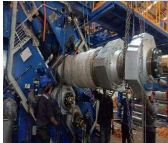
Lifting and setting of steel calendar machine at Gajah Tunggal Project
